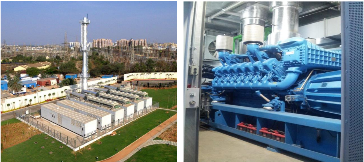
Figure 6. Rotary UPS systems installed at NetApp-Bangalore data center. The system has a built-in flywheel for energy storage and supply.
