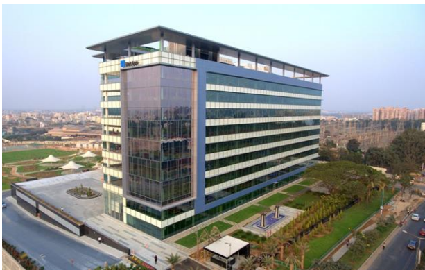
Figure 1. NetApp Bangalore campus, including lab and data center
